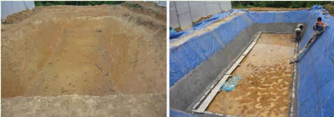
Lining of tank for rain water harvesting
