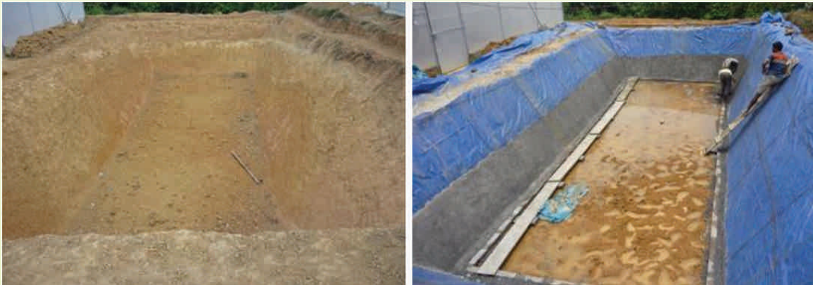
Lining of tank for rain water harvesting
